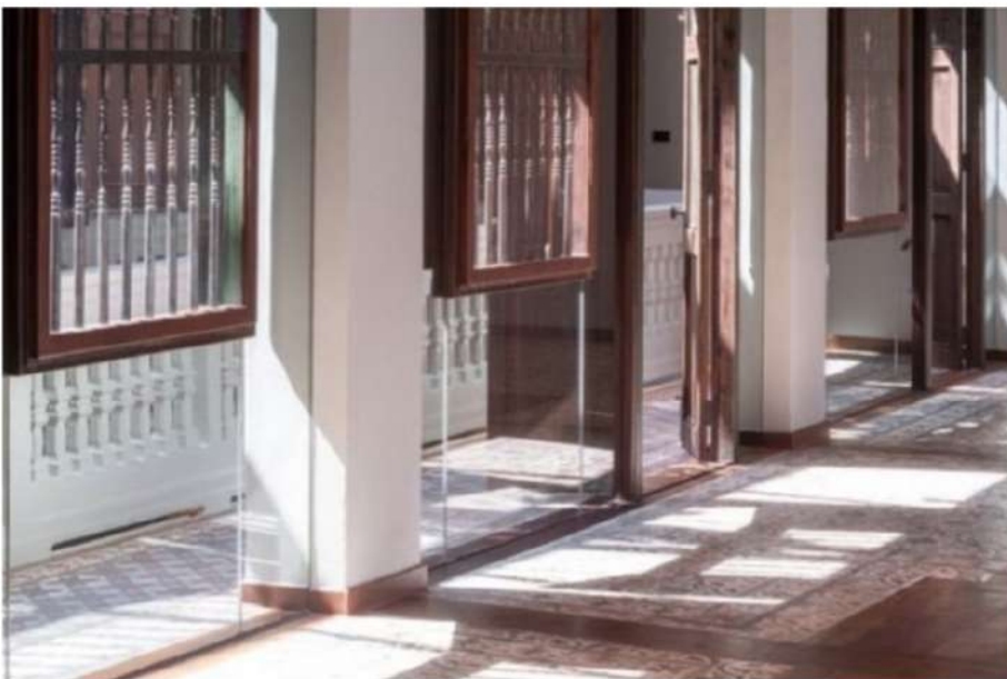
Figure 8 The designers decided to restore old windows and doors to new glass walls and kept the antique floor tiles after realizing their authenticity through VERNADOC drawings. (Photo: www.baantrok.com )
