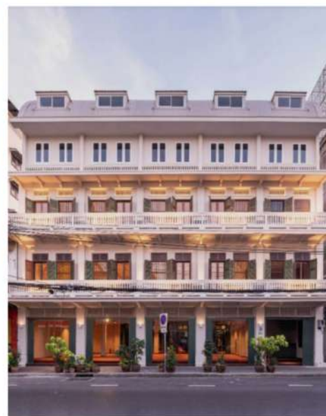
Figure 2 Baan Trok Tua Ngork after the renovation, 2022.
