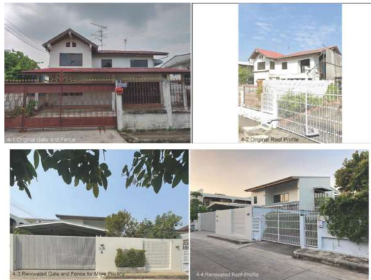
Figure 4: Comparison of Original and Renovated Exterior
